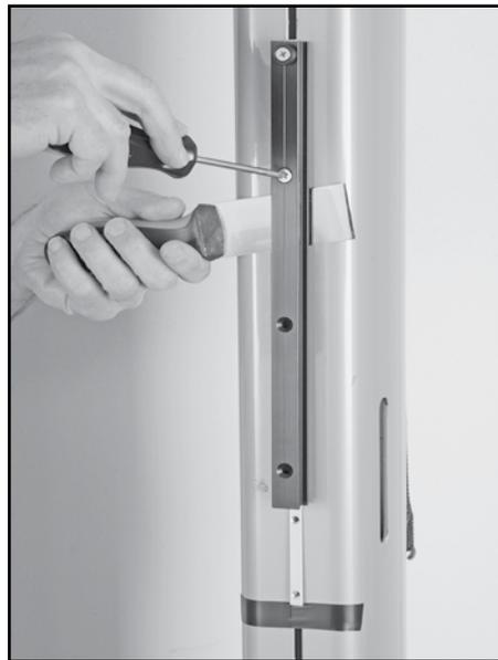
Slide slugs into place with putty knife. Loosely install 5 mm x 20 mm screws.
