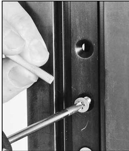
Remove plastic locator screw and replace with mounting screw. Use blue Loctite adhesive.
