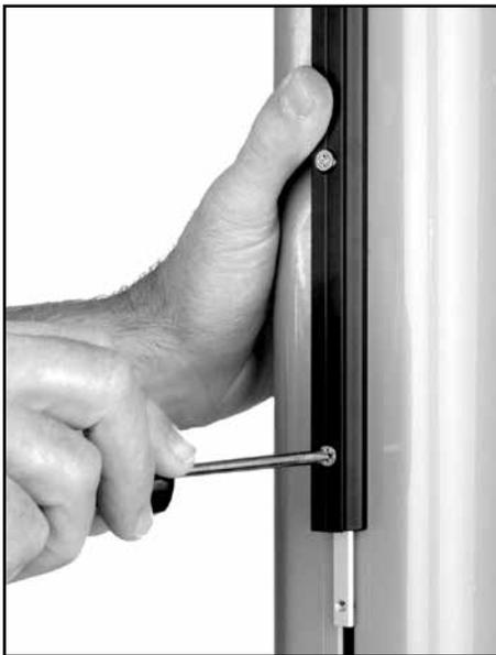
Loosen top screw. Slide top track up and position next 2.05 m (6'8 7/8") track.
