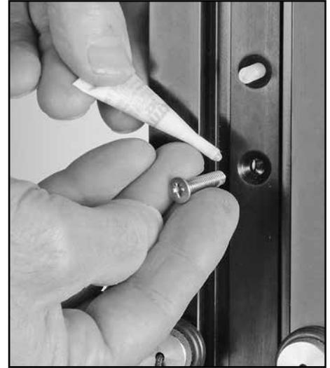
Install screw in open slug hole using blue Loctite adhesive.
