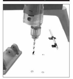
Drill into cabintop and clean any drilling dust from holes.
