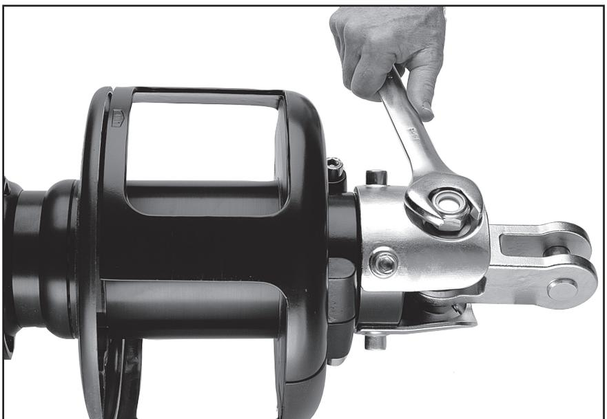
Determine height of link plates to provide anchor clearance and cut to length.
