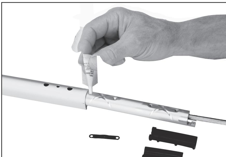
Hold plastic wedge in place with thumb as you insert into foil. Line foil holes with connector screw holes.
